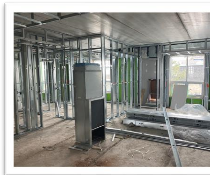
Building B – Second floor CFS and precast walls complete
